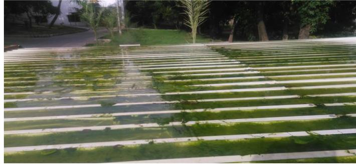
**Fig 3 The surface of the slope showing luxuriant growth of algae**
