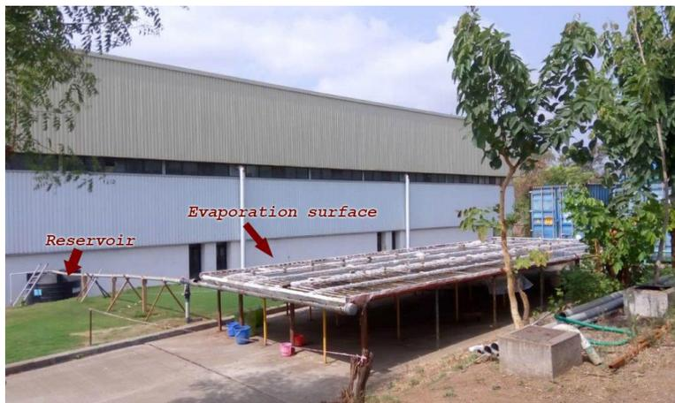
Fig 2 Slope tank system for evaporation of R/O reject
